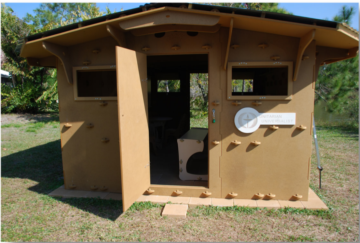
Terrapeg House, Shelter In A Day
