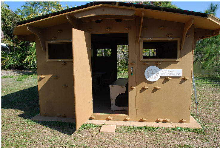
Doors and windows with locks and screens
